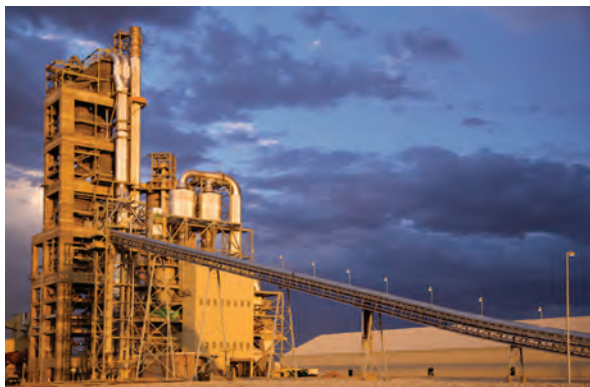
Figure 1-4. Portland cement manufacturing plant (Courtesy of GCC).
