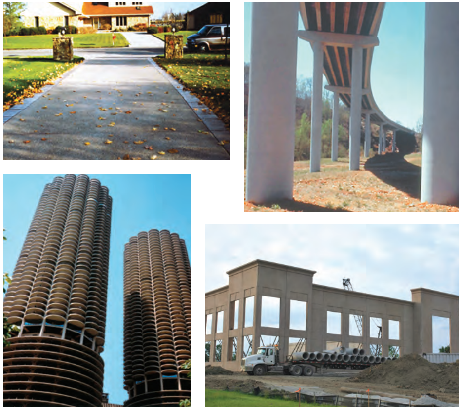
Figure 1-9. Concrete's primary markets include: pavements, bridges, and high-rise and low-rise buildings.
