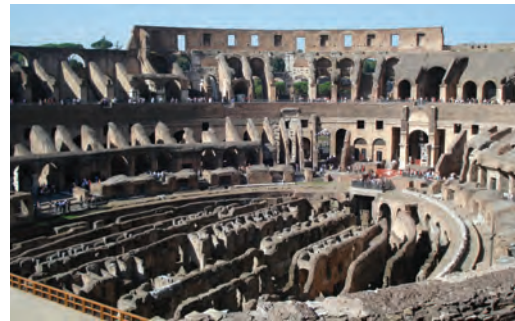
Figure 1-10. Coliseum in Rome, completed in 80 AD, was constructed of concrete. Much of it still stands today (Courtesy of J. Catella).
