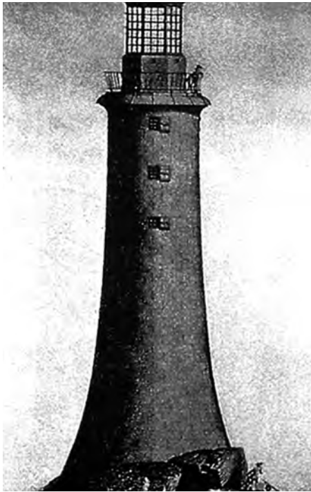
Figure 1-11. Eddystone lighthouse constructed of natural cement by John Smeaton.
